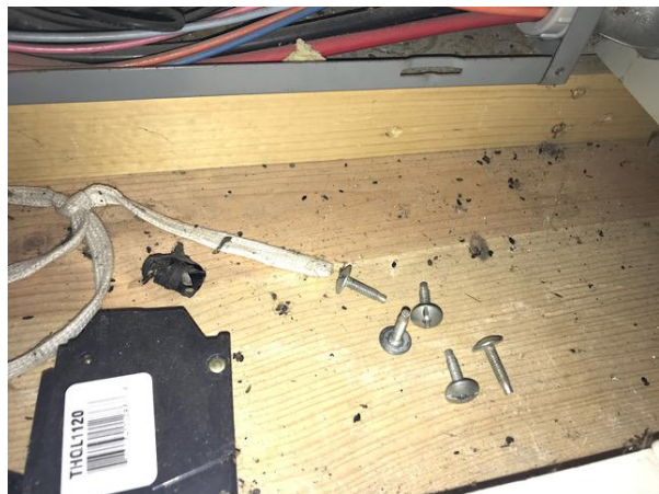
Rodent droppings present below the electric panels
