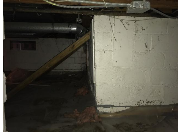
Leaning portion of north foundation block wall. Have evaluated by a structural engineer.
