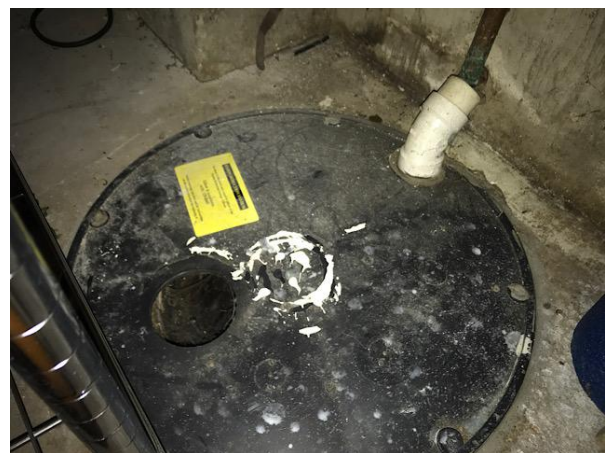
Sump pit is not sealed for Radon
