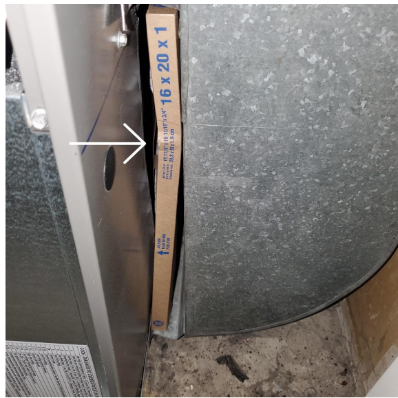
Unsealed furnace filter opening
