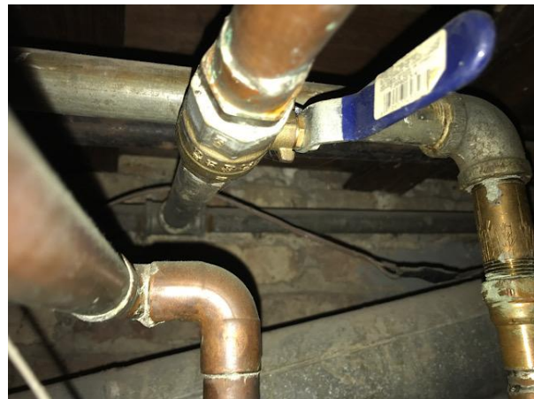
corrosion: missing dielectric union
