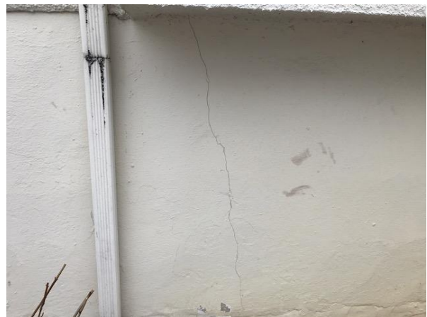
Cracks in foundation walls visible from the exterior
