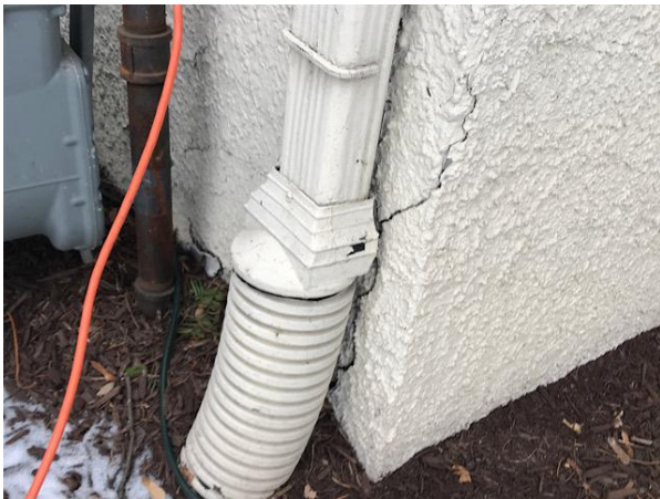
Example of cracks in stucco siding
