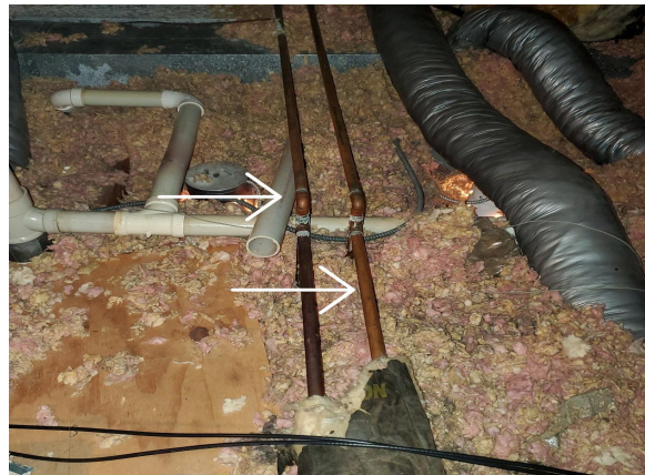
Exposed active water lines in attic
