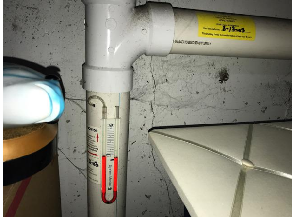
Interior Radon vent pipes
