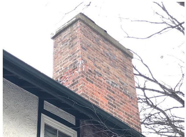
Spalled bricks & cracked cap
