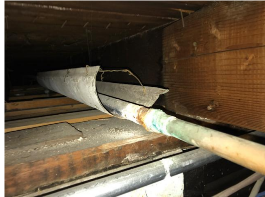
Rusted / Corroded copper to galvanized pipe unions. Missing several dielectric connectors
