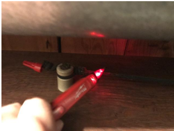
Live knob and tube wire present in the basement and east crawl space
