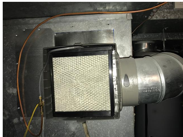
Humidifier is damaged and dismantled
