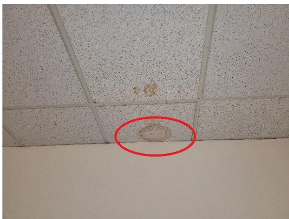
Active water leak in basement family room
