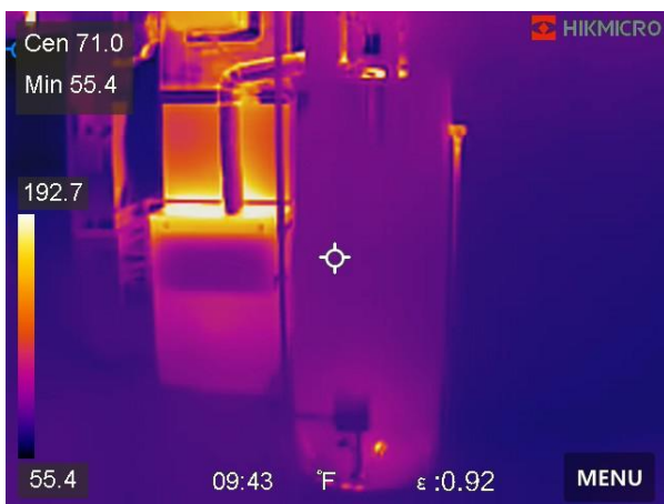
Thermal image of furnace & water heater
