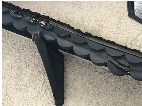
Multiple layers of shingles. Damaged tabs. Rotted fascia boards
