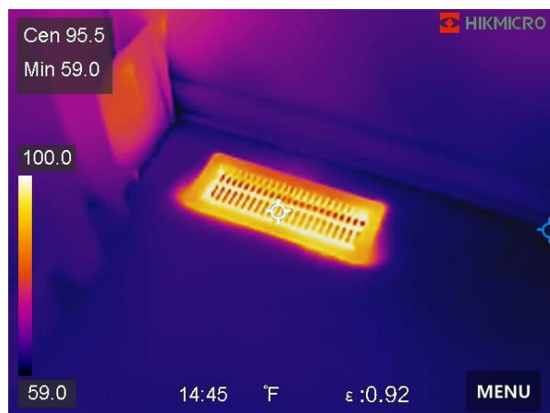
Infrared image of active heating duct
