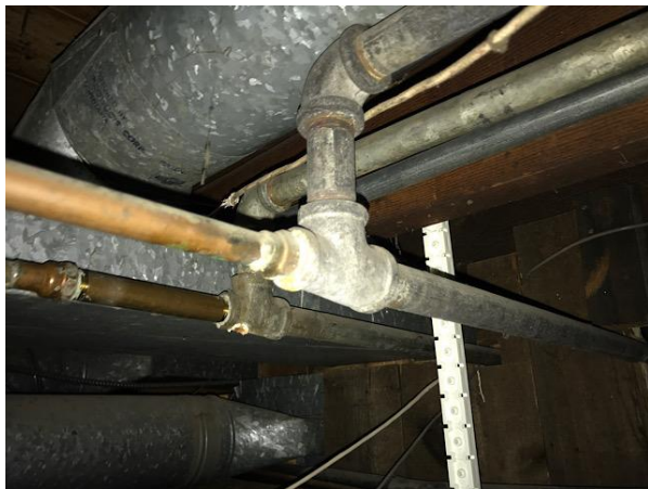
corrosion: missing dielectric union
