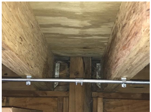
Water stains inside garage, below the roof deck
