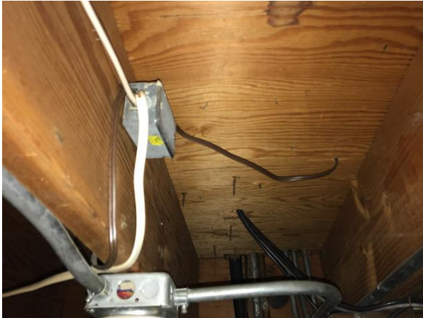
Brown, lightweight, lamp cord wires improperly routed through the floor
