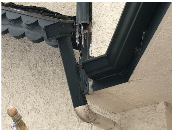
Loose front gutter and downspout
