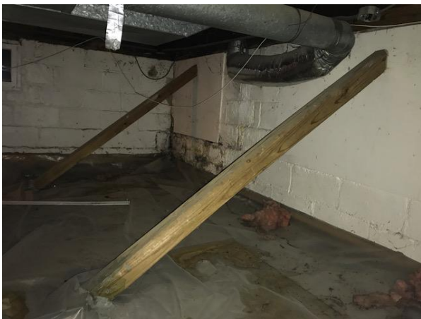
Poorly supported with 4x4 posts
