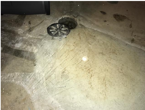
Utility sink water backing up through the floor drain
